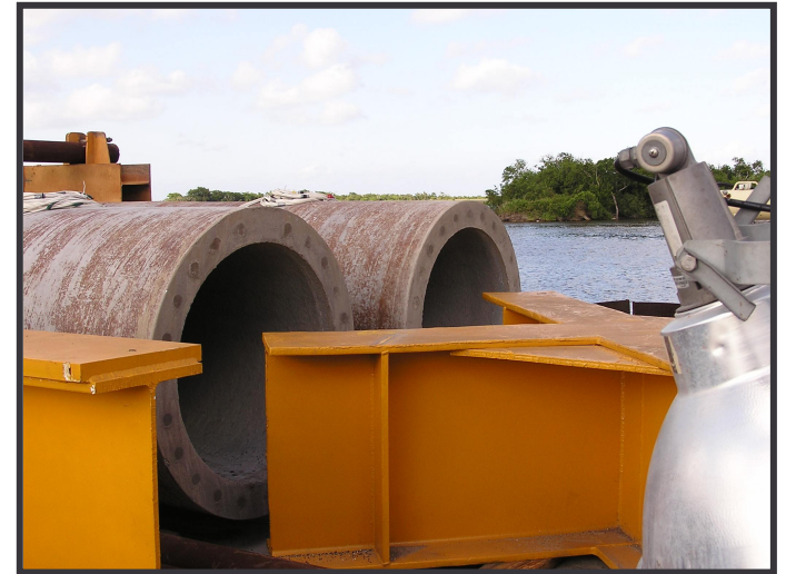
Concrete Test Pile segments waiting for placement ↓
