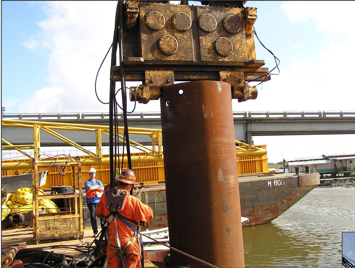
↑ Test Pile casing being placed near Leeville Bridge
