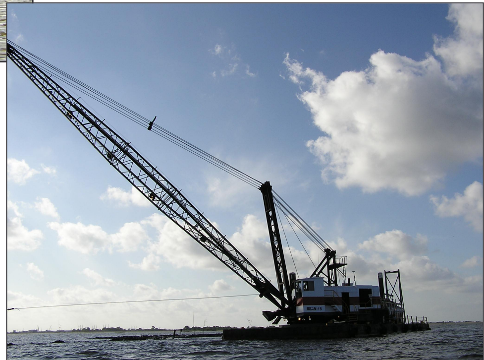
←↑ Dredging operations for the Test Pile Program.
