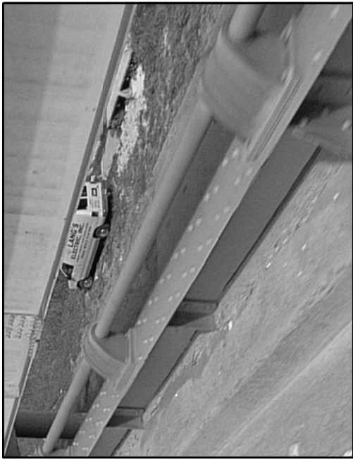
EXISTING STEEL BRIDGE RAIL W/ ALUMINUM RAIL
